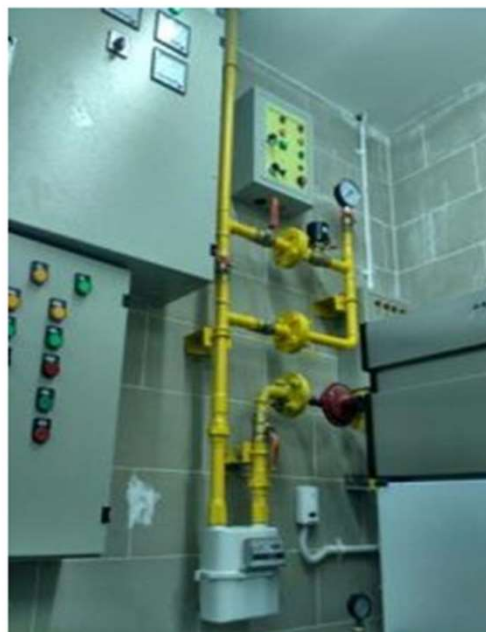
Instalasi Pipa Gas
