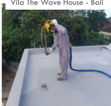
Coating Area Rooftop Vila The Wave House - Bali
