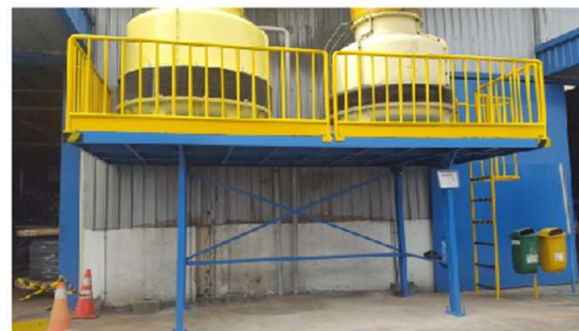
Instalasi Cooling Tower dan Safety Support
