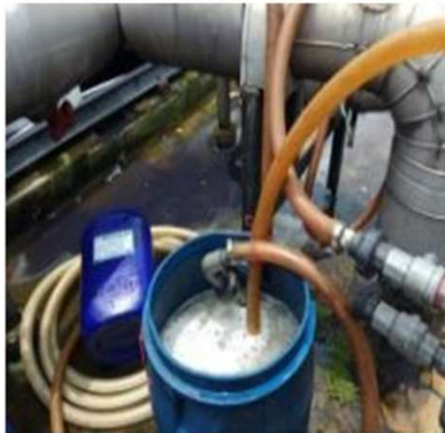
Descaling dan Cleaning Chiller
