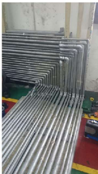
Relokasi Pipa Oil Cooler
