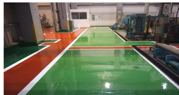
Coating Lantai Epoxy
