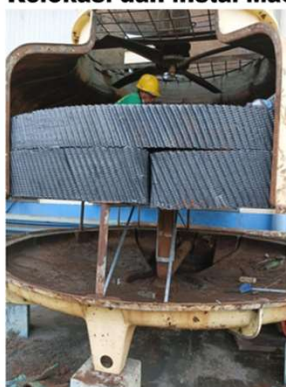
Penggantian Spare Part Cooling Tower
